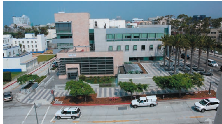
3 Environmentally friendly buildings. Santa Monica (California)
