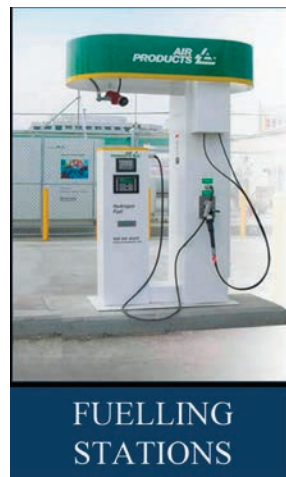
1 Prototype of H2 fueling station, Santa Monica (LA)
