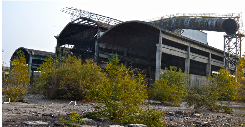
Lucchini Ex-mill Production Building
