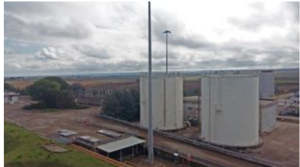
Figura 4 Campomarino water tanks
