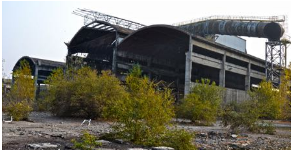
Lucchini Ex-mill Production Building
